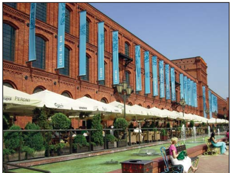
Manufactura in Lodz-from factory to downtown mall.
