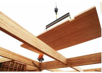
SmartLam Cross Laminated Timber Panels
