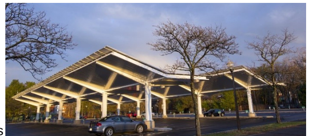
Solar PV Carports at University of Massachusetts
