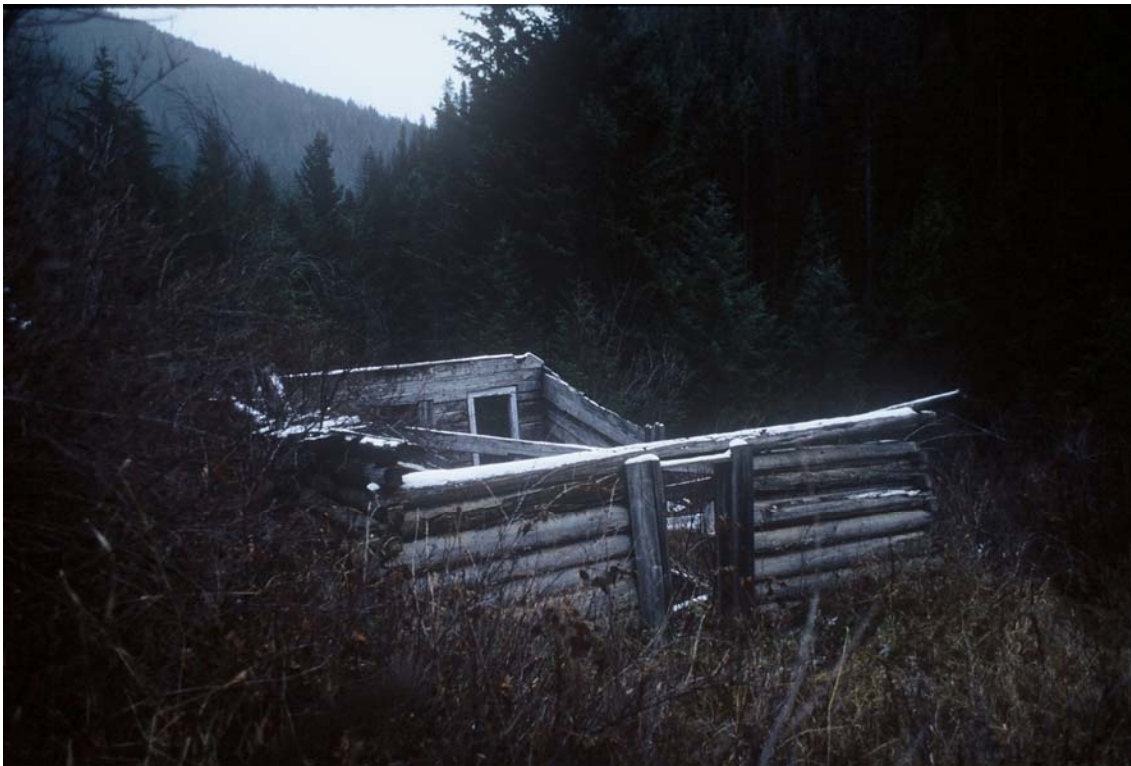
Figure 6. Cinkers/Louiseville Structure 3, possibly Log Saloon. Photo taken during 1995 Field Season by T. Light.
