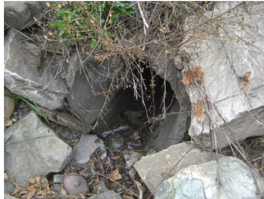
University of Montana West Outfall Location: 46.866459, -113.984491
