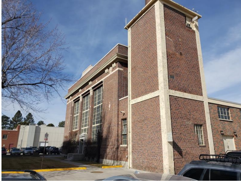
Figure 3-1: UM Current Heating Plant Building
