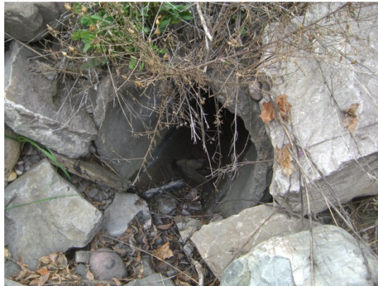
University of Montana West Outfall Location: 46.866459, -113.984491
