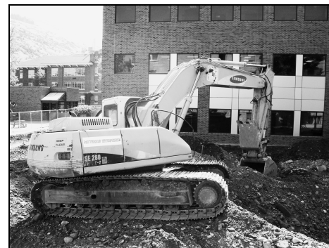
Phase II: Back hoe in action, taken from the South exit
