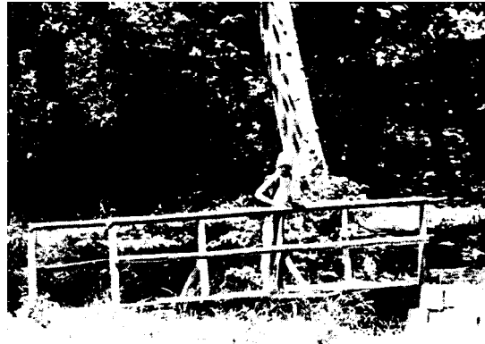
Figure 8. --Onsite management includes modifications, such as bridges, which can vary from simple logs for foot travel to complex developments capable of supporting automobiles.
