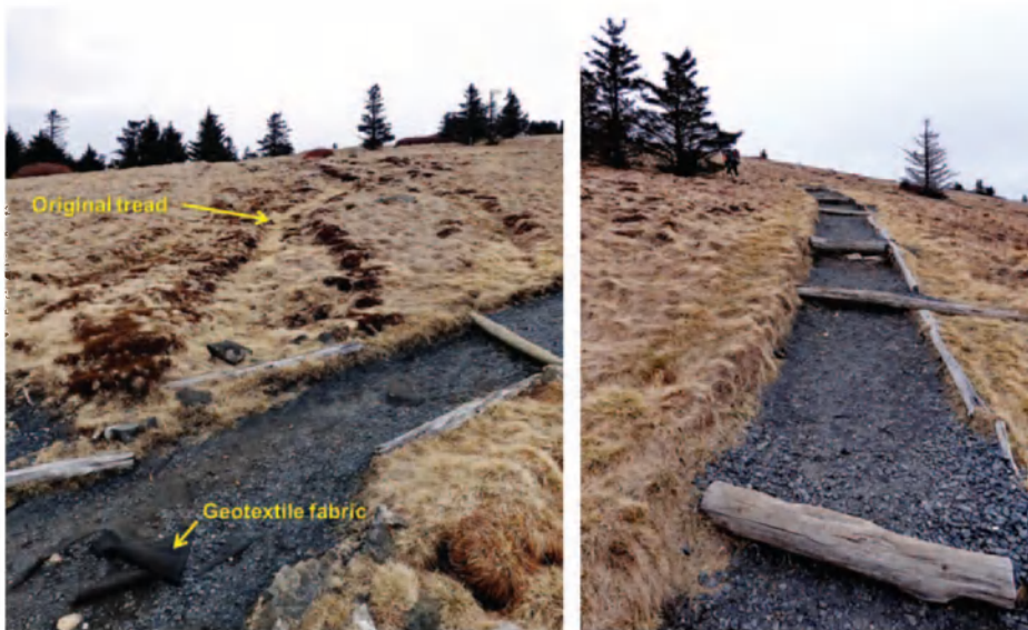
Figure 6. Restoration of a steep “fall-line” segment of the Appalachian Trail (left) in the popular Roan Highlands area of North Carolina. Restoration work conducted in 2001 included laying native sod excavated from the new side-hill alignment (right) and temporary fencing to discourage use. Geotextile fabric and cellular confinement materials were used, but both surfaced after displacement of the applied gravel. Premixing gravel with native soils is a more natural and sustainable practice.
