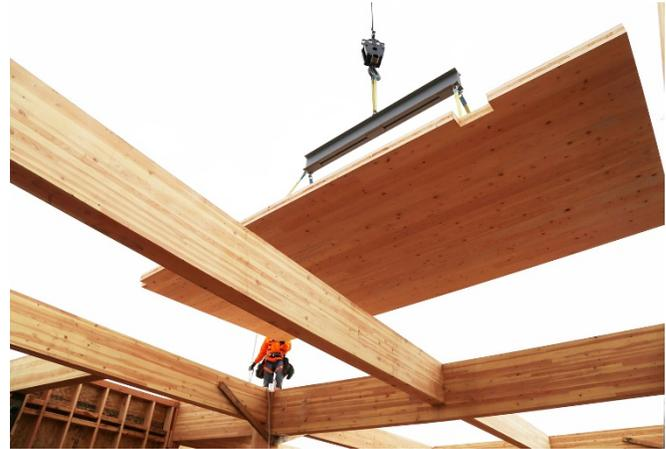
SmartLam Cross Laminated Timber Panels
