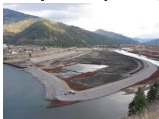
November 2007 (bypass channel near completion)
