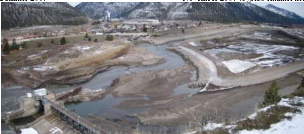
March 28, 2008: Milltown Dam and Reservoir within hours of breaching of cofferdam
