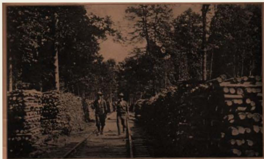
BARKED WIRE STAKES, TO BE USED LATER AT THE FRONT, CUT AND STACKED ALONG BROAD GAUGE RAILWAY IN A HARDWOOD FOREST IN CENTRAL FRANCE
