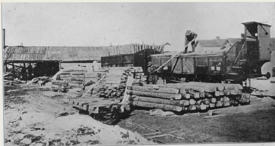
20th ENGINEERS LOADING LUMBER AND TIES ON FRENCH CARS. THE CAR AT THE LEFT IS LOADED WITH BARBED WIRE STAKES. THE BUILDING AT THE END OF THE RIGHT-HAND CAR CORRESPONDS TO AN AMERICAN CABOOSE
