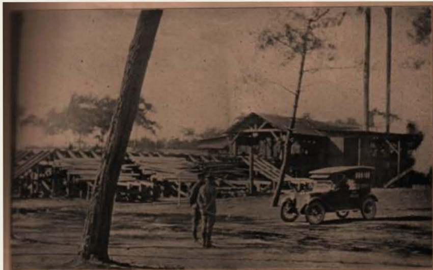
AMERICAN 20" SAWMILL NEAR PONTSEIX, LANDES. COL. BENEDICT WITH HIS BACK TURNED, IN THE FOREGROUND, STANDING NEAR NARROW GAUGE TRACK OVER WHICH LUMBER IS TRANSPORTED THREE MILES TO THE SHIPPING YARD.
