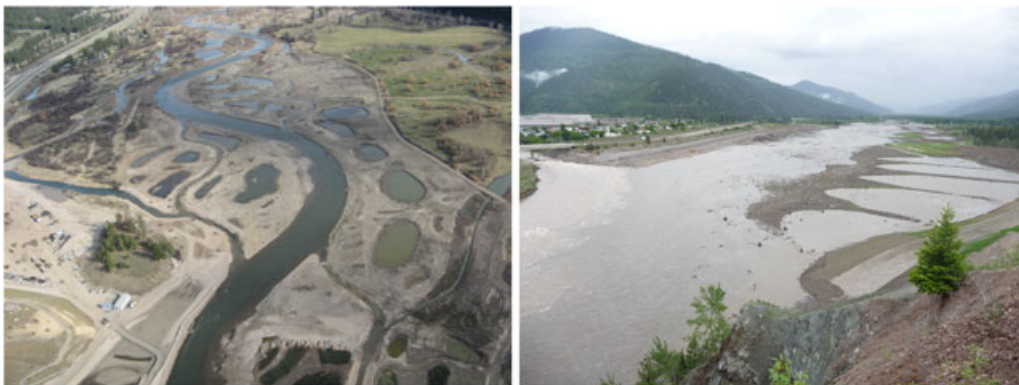
Figure 10. Milltown restoration reach. Left image shows newly constructed channel in April 2011 (courtesy of G. Matson); right image shows restoration reach in June 2011 at high flows; former Milltown Dam site is in lower left (courtesy of J. Bean). This figure is available in colour online at wileyonlinelibrary.com/journal/espl
